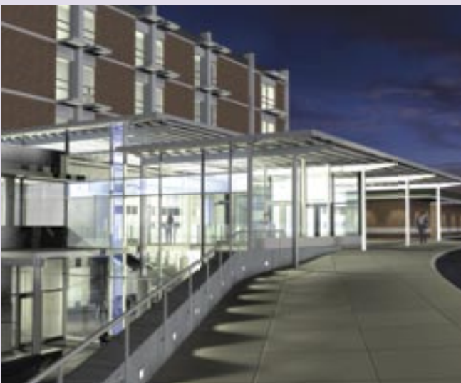
Designed to be wheelchair accessible, the east entrance will be the main point of entry for patients and visitors to Diagnostic Imaging, Cardiac Diagnostics, the Ambulatory Care Unit and admitting.
